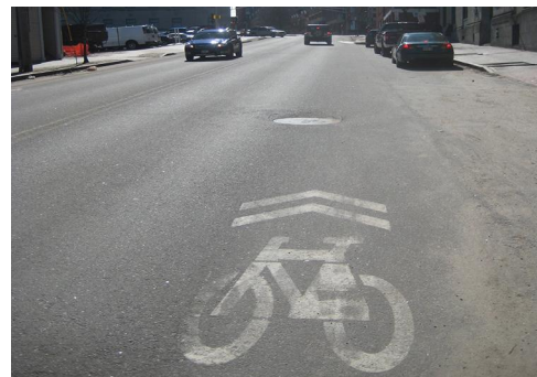
Example of a Sharrow paint marking on Congress Avenue in Portland where bicyclists and vehicles share the same travel lane
